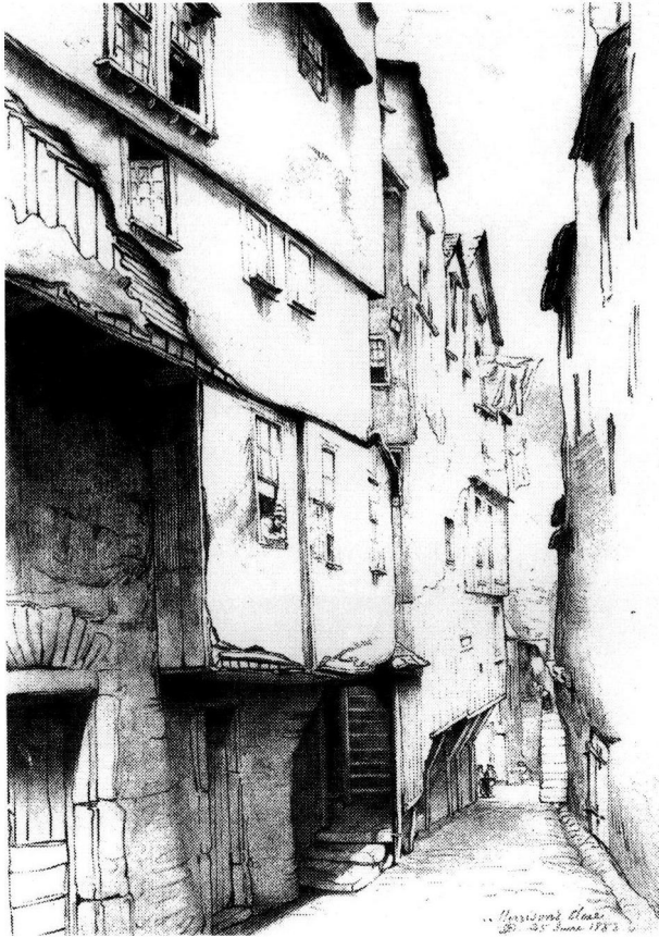
Figure 5 'Morrison's Close, 117 High Street, Edinburgh. 1853' showing multi-storey timber-clad dwellings, some covered with a later lime render Reproduced courtesy of RCAHMS
